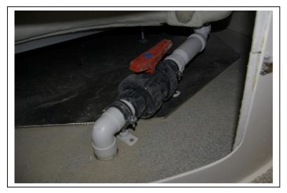
The straight-through trap should PRECEED the valve in the pipework. It may be the case that this is not possible and the trap has to be positioned further down the line, even in the ceiling void of the room below.
